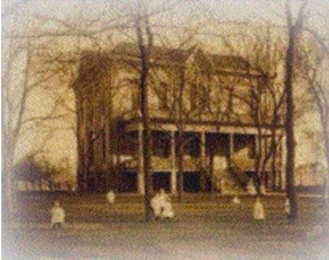
Building before renovations
