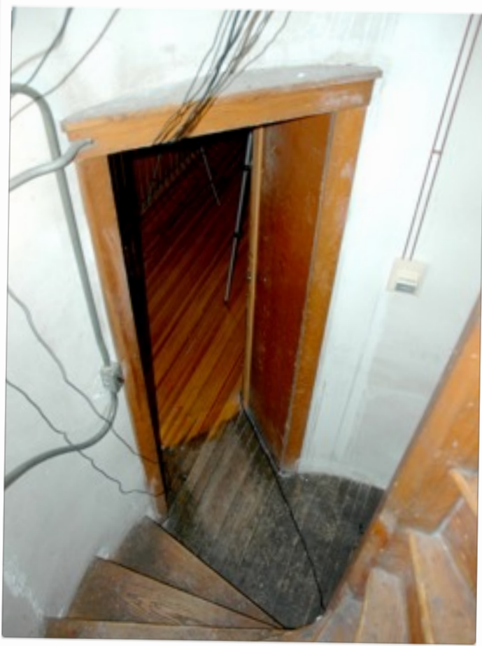
The tower stairs looking down at the organ practice room
