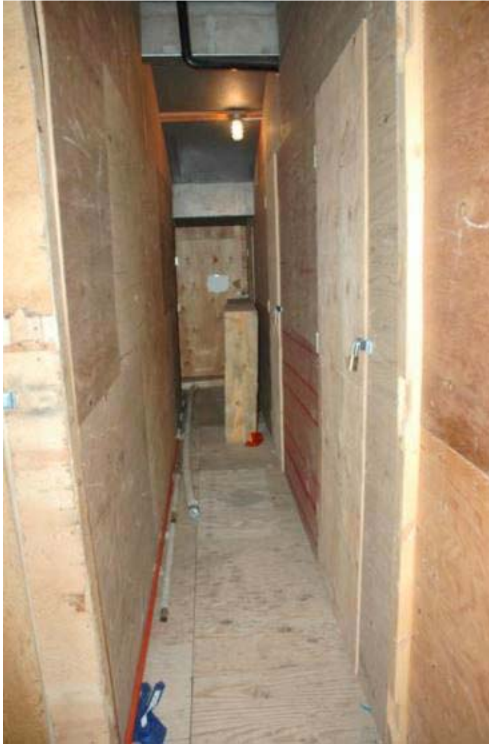
Hall leading to the storage area
