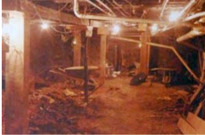
The Bar during renovations (1991)
