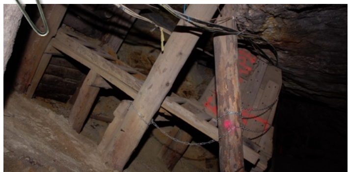
Broken Timbers from past collapses
