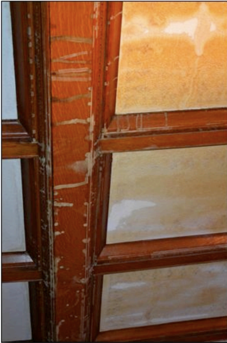
Water damage on the ceiling in the main entrance room
